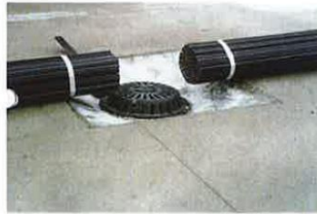
Problem-free Direct Placement on Concrete Surfaces (International Stadium Yokohama)
