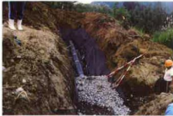
Soil-and-Water Conservation Works
