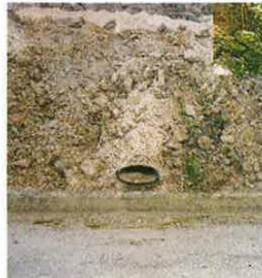
Solution to Clogging (photo showing clogging by inadequate resistance to pressure)
