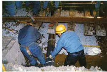
Railroads (demonstrating resistance to heavy loads imposed by train movement)
