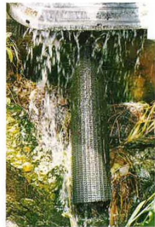
Solution to Clogging (photo showing clogging of non-continuous water collection openings by organic and other elements brought on as a result of worsening water contamination of recent years)
