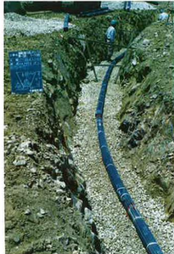
Mitsuba Drain Installed for Underground Drainage
