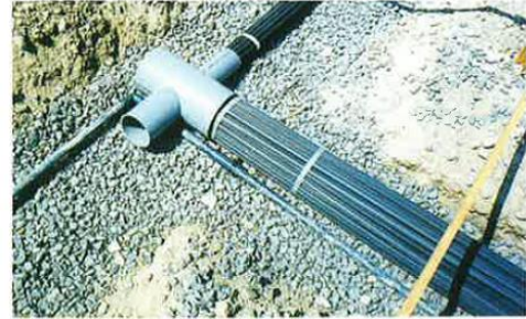
Coupling Joint Designed and Made to Meet Specific Needs of a Particular Site
