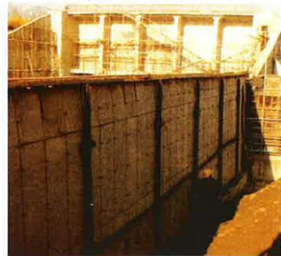
Drainage along the Back of a Structure
