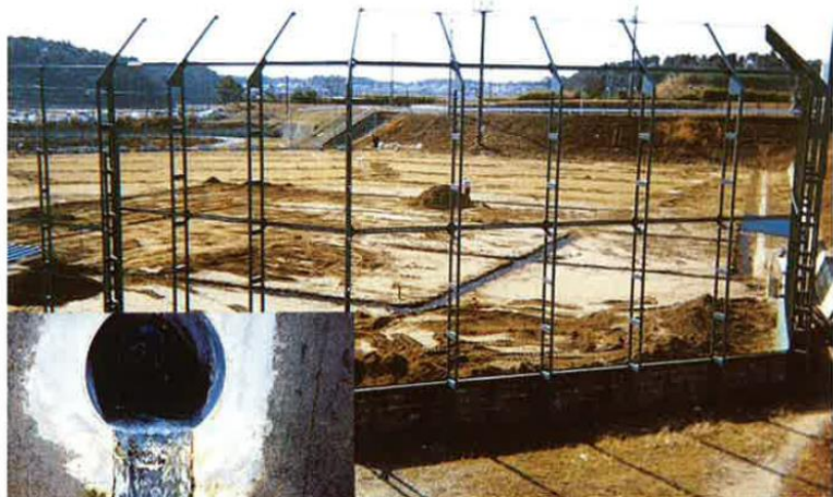
Subsurface Drainage through Culverts under School Grounds
